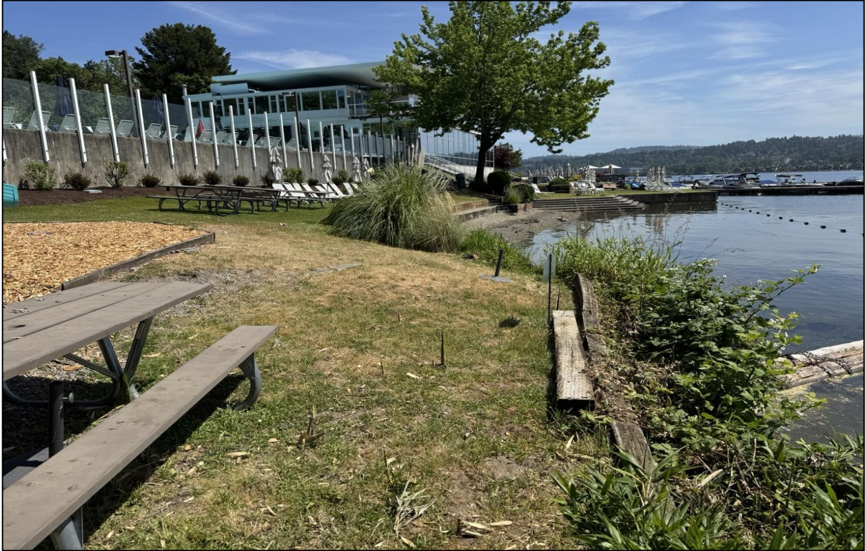
Photo 5. Northeastern overview of proposed rockery and retaining wall improvement location.
