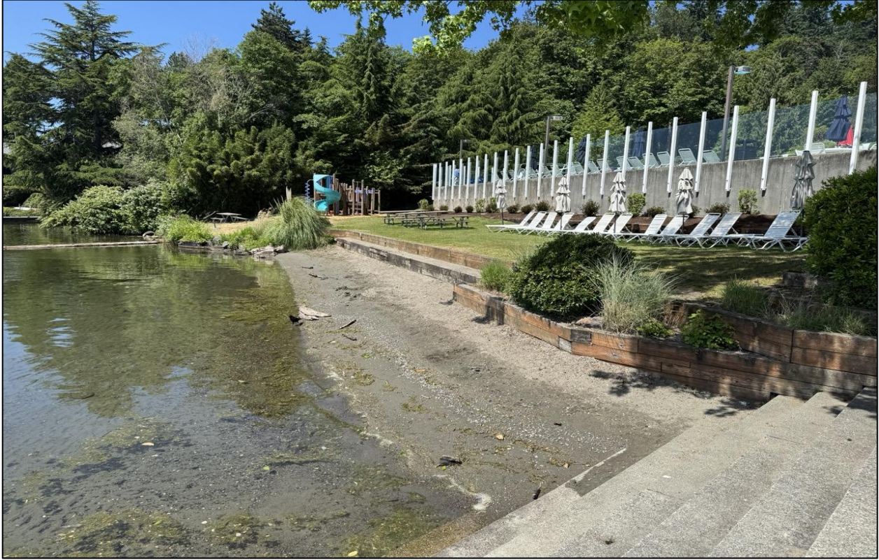
Photo 6. Southwestern overview of proposed rockery and retaining wall improvement location.
